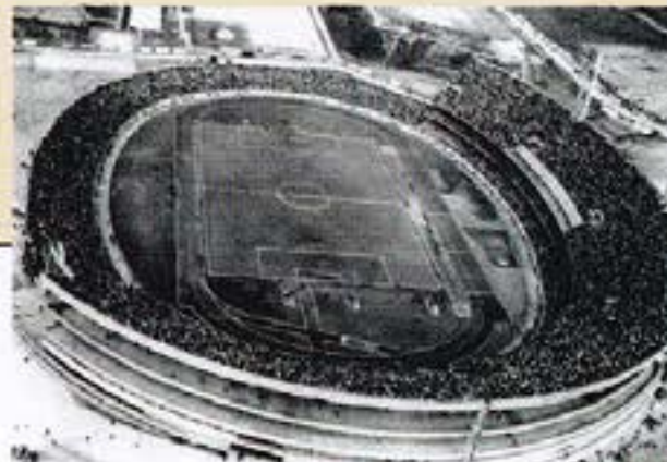
After its opening in 1960, still with the superior ring incomplete
